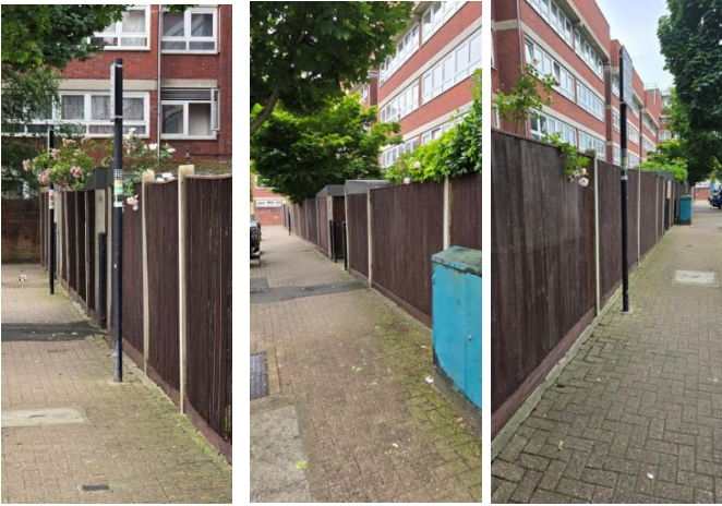
Photos of the repaired/repainted fencing on Shuttleworth Road
